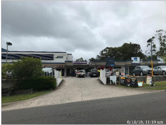
Complex front external elevation
